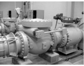
Standard with Rubber Disc Seats and Stainless Steel Body Seats, Crispin **Swing Checks are ideal for aggressive** water and sewage applications.
